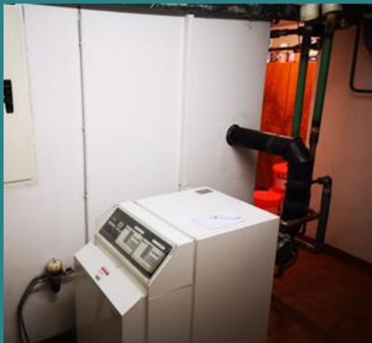
Old oil boiler (left) and new pellet system (right)
