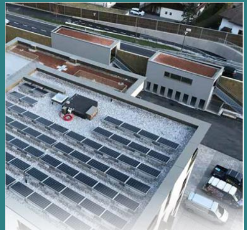
PV modules are installed at a part of the flat roofs, the other part is covered by terraces
