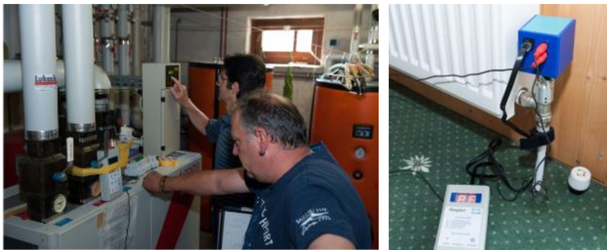
Figure 3: Installers performing a boiler check measures and hydraulic balancing equipment installed at a radiator valve 14
