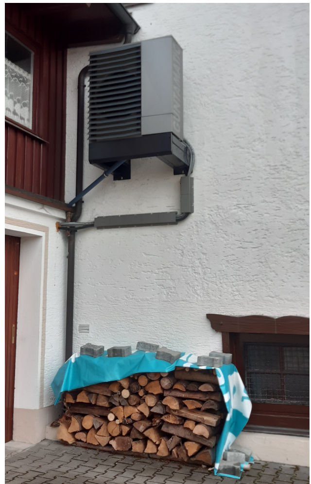
Heat pump installed on the wall of a house and storage of logwood on the floor
