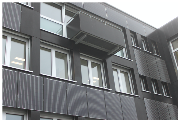
Photovoltaic panels integrated in the façade of a building
