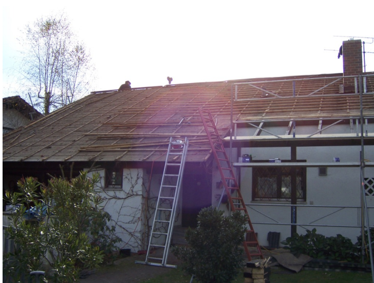
Refurbishment works for insulation of the rooftop of a single-family house
