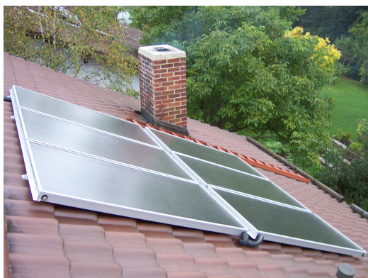
Solar thermal collectors installed on the roof of a single-family house
