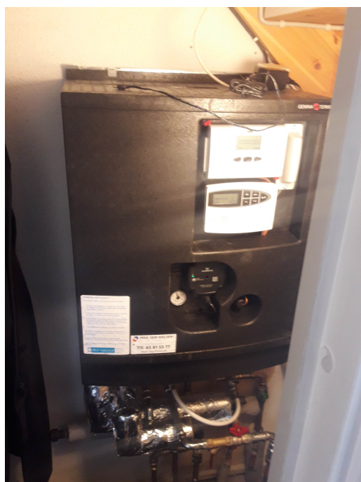
Building's connection to a district heating network with a heat exchanger
