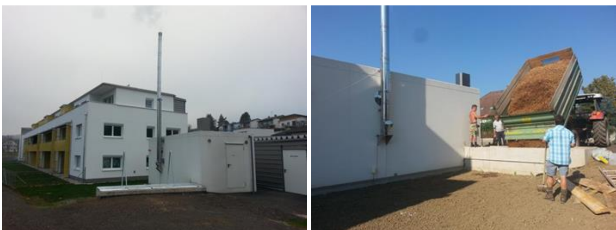
Figure 10 Example of a realized biomass micro grid heating container, heating blocks of flats
