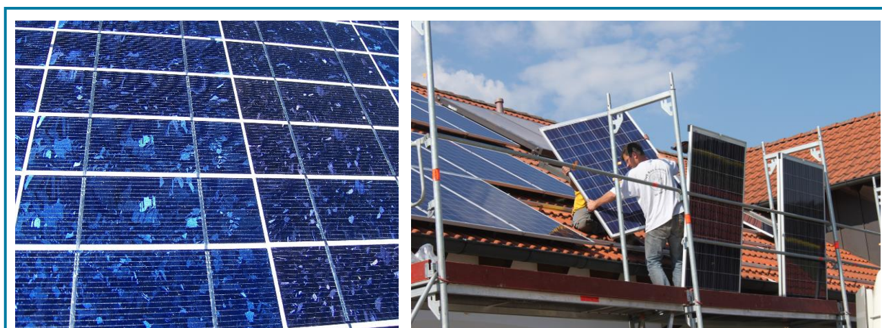
Figure 20 PVs for heating - cell and installation
