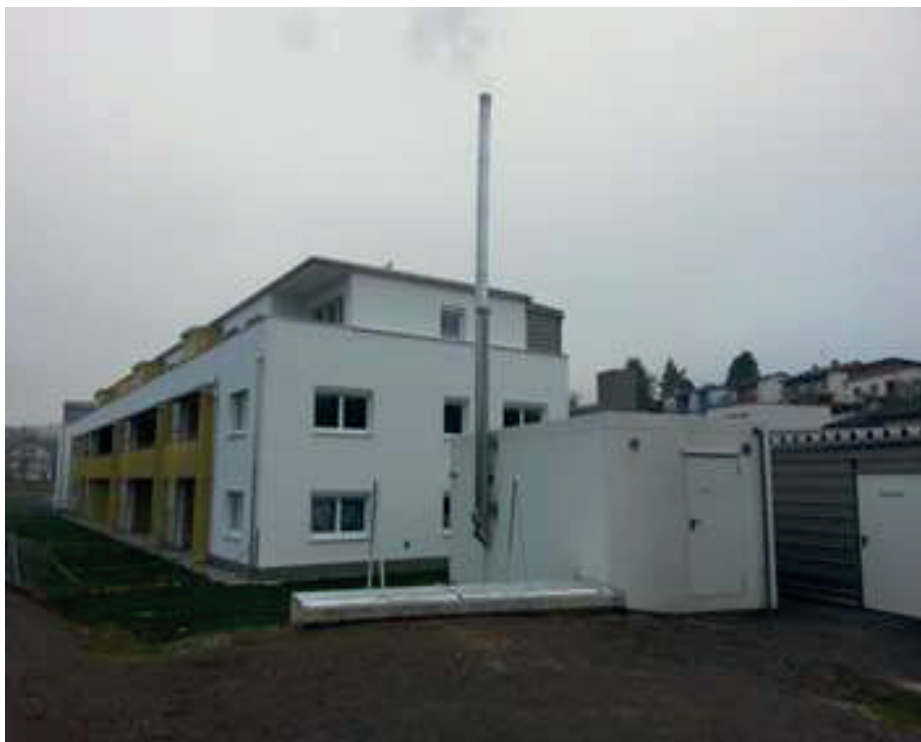
Example of a realized biomass micro grid heating container, heating blocks of flats
