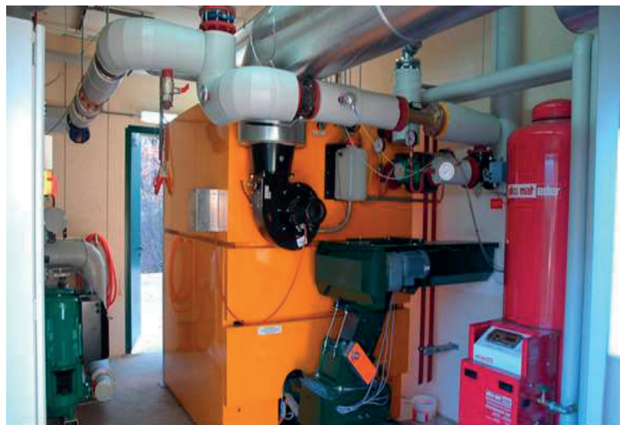
Interior of a biomass micro grid heating container
