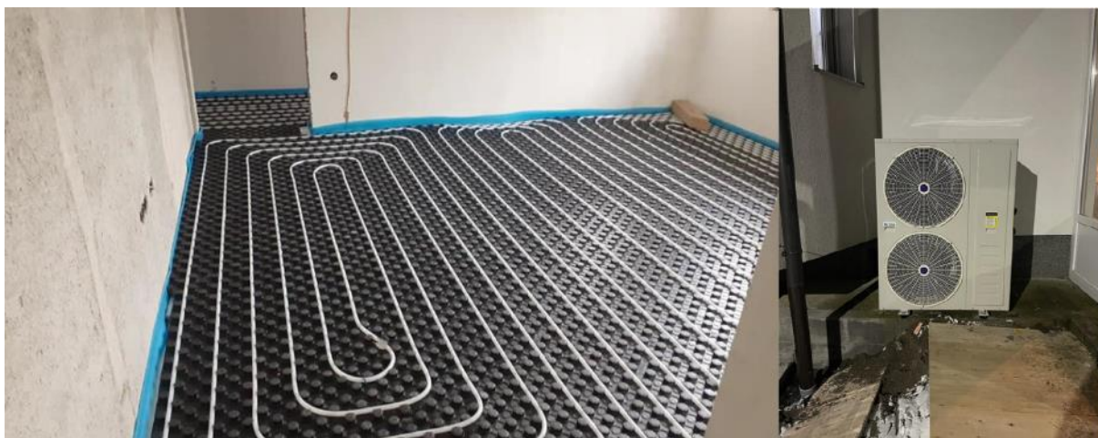
Figure 9: Installation of underfloor heating and heat pump
