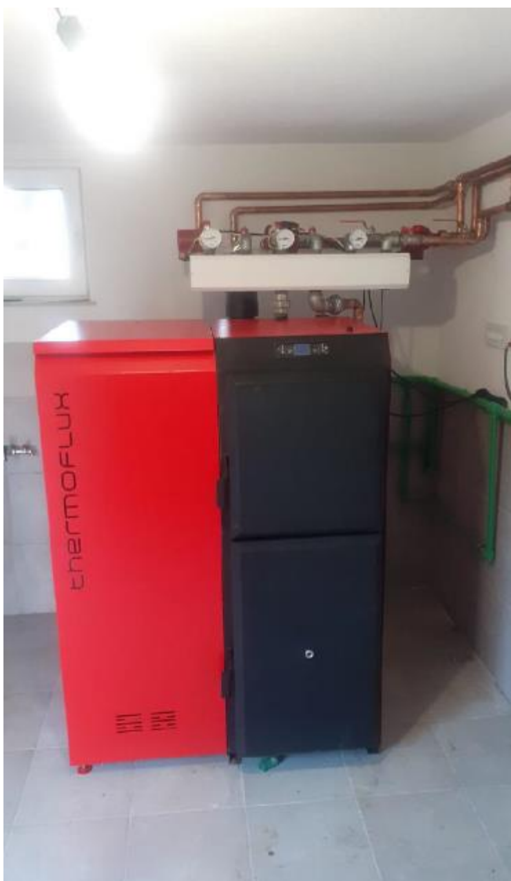
Figure 5: New pellet boiler
