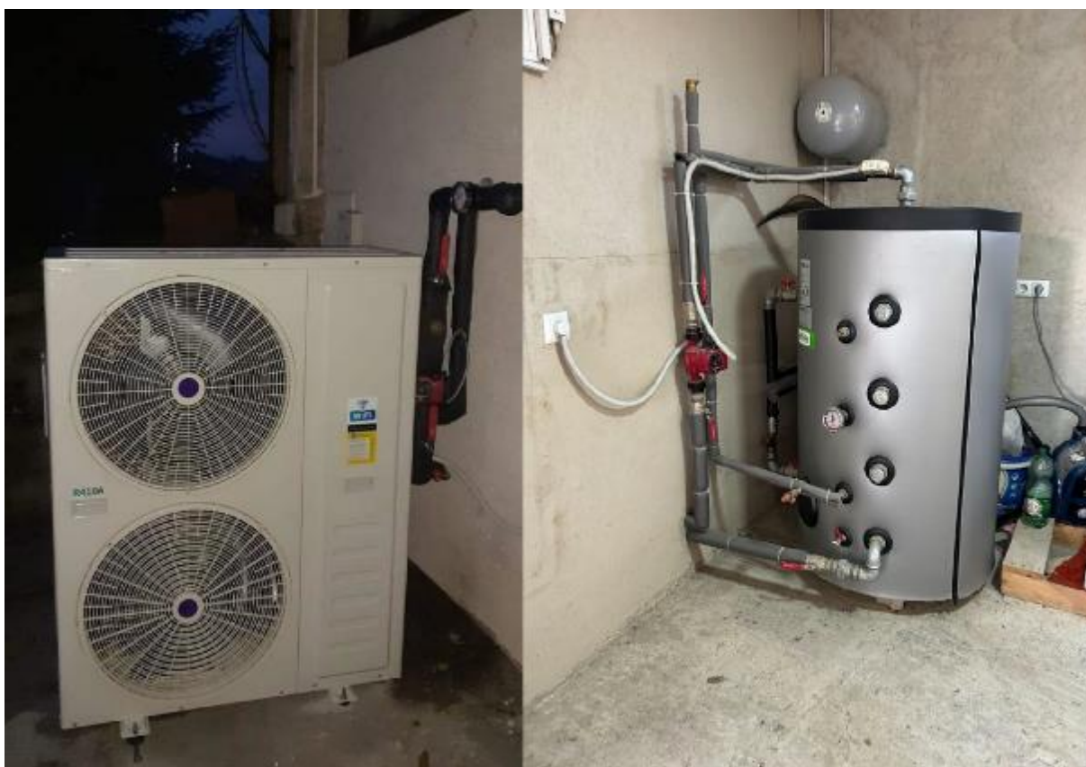
Figure 10: Installation of the second heating pump with buffer
